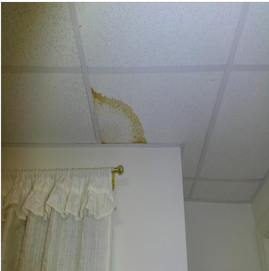
Image Number: 35 Observation: Moisture stains were observed within the interior at a closet and office. Cause: It was determined that the condensation from the plumbing pipe is causing this water pattern and damage. Remedy: Contact a licensed plumber to determine a remedy for this issue.
