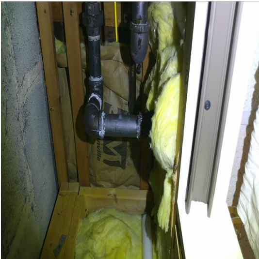
Image Number: 36 Observation: Moisture stains were observed within the interior at a closet and office. Cause: It was determined that the condensation from the plumbing pipe is causing this water pattern and damage. Remedy: Contact a licensed plumber to determine a remedy for this issue.
